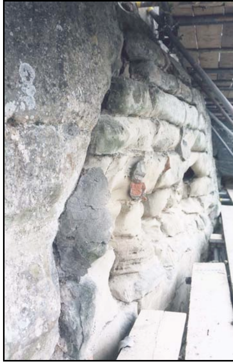
Plate x: erosion of sedimentary stone at Warwick Castle
