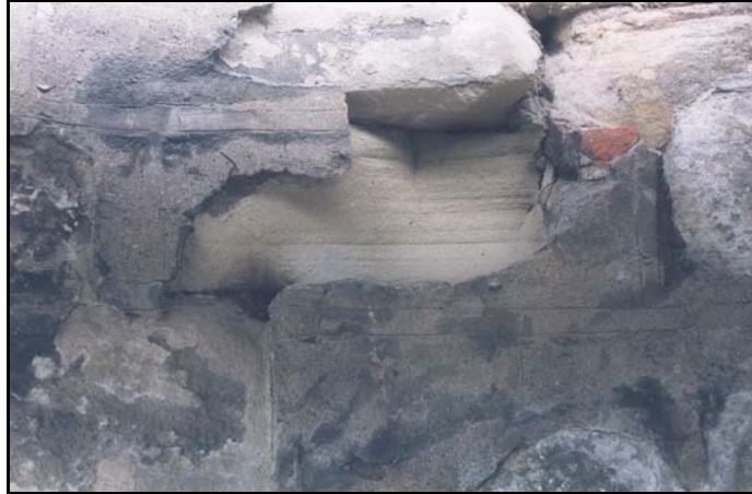
Plate x: erosion of sedimentary stone at Warwick Castle
